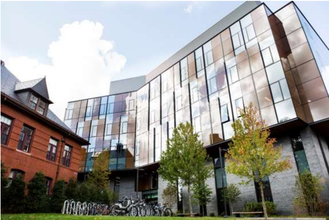
The new Science and Engineering Complex (SEC), September 27, 2017
